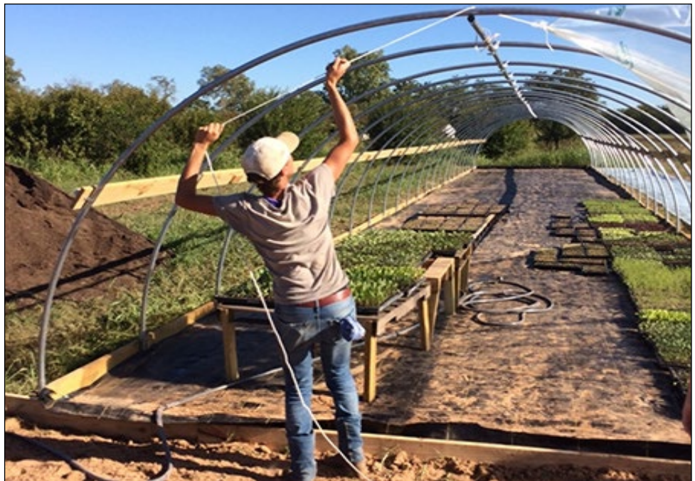
Building a hoop house at Farmshare Austin
